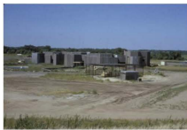
The African Veldt, seen here during construction, opened in 1972
